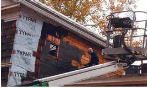
Removing old dilapidated shingles and rotted millwork on the west side of Cooper - Ferry gallery over studio.
