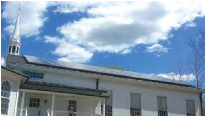
On the roof of the First Congregational Church of Old Lyme are 136 solar panels which reduce the cost of electricity, as well as reduce the environmental footprint of the church.
